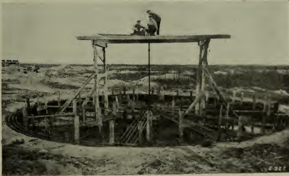
REINFORCEMENT OF THE BASE OF ONE OF THE PYLONS.
